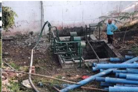
Digester Outlet Sump
