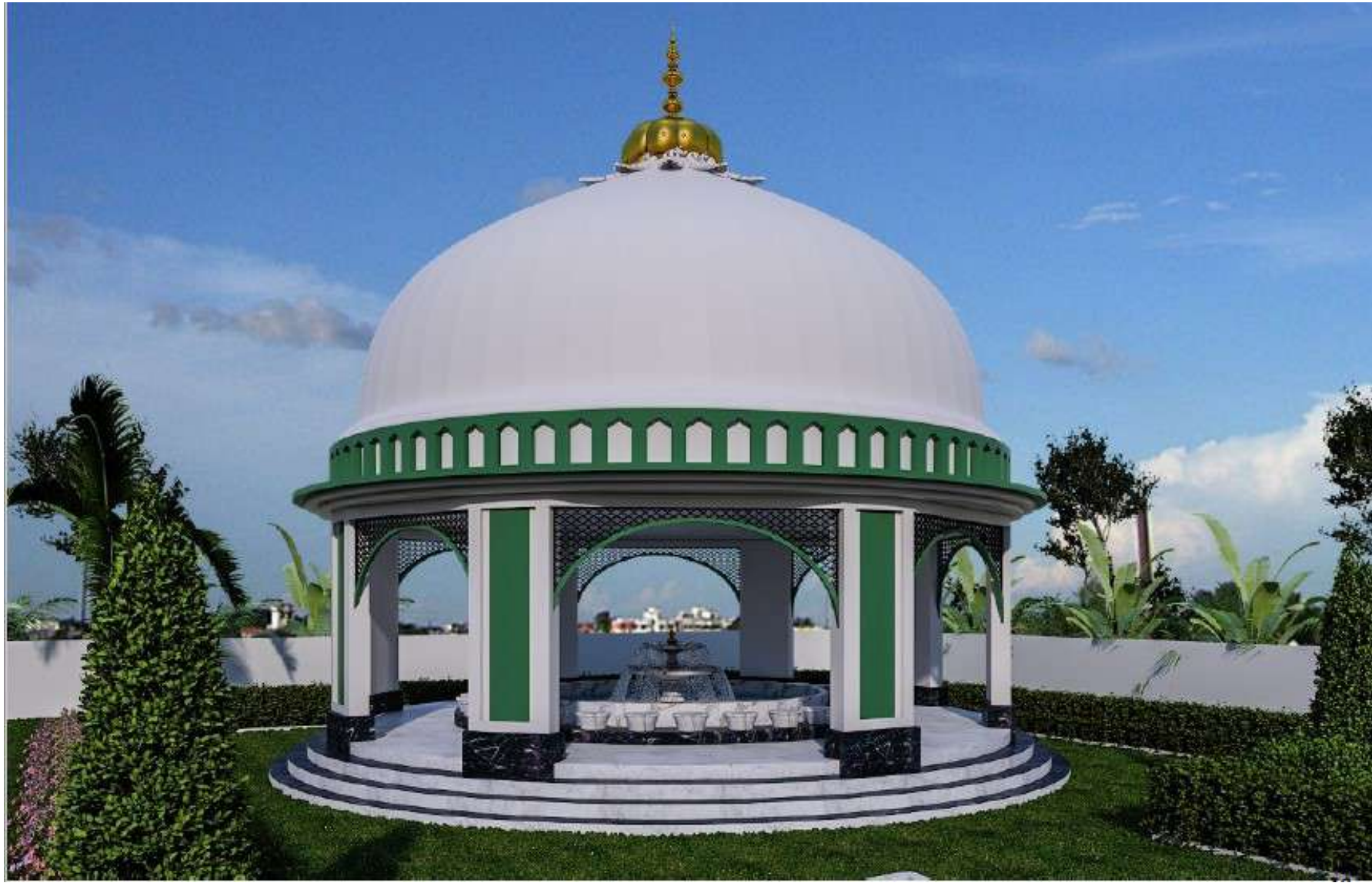
Typical architectural view of Choto Ujkhana
